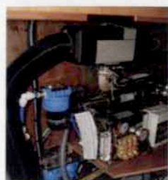
ABOVE: Excellent access to the 'technical room'
